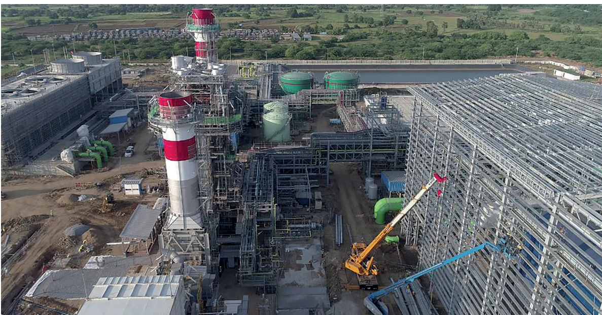
The plant under construction
